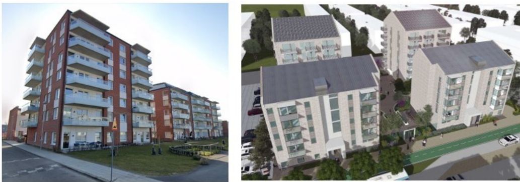
Figure 16. Building blocks before implementation of construction project (Left) and render of newly constructed blocks post-implementation (Right)
